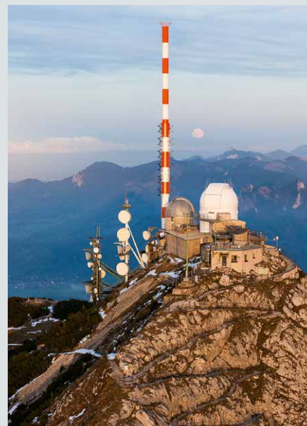
The Wendelstein transmitter is one of the test transmitters for 5G broadcasting mode FeMBMS.
